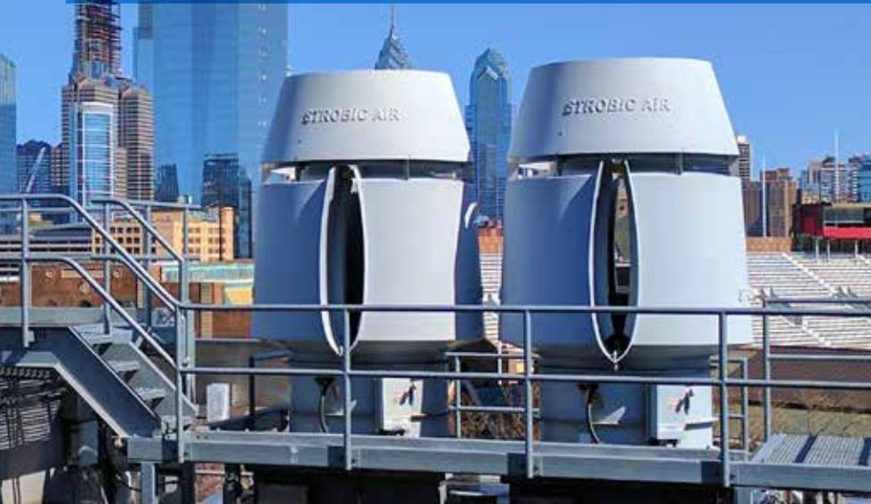
A life science building in Boston with Gold status LEED certification was looking to aggressively drive energy savings. They installed SmartStack™ to monitor four large high plume lab exhaust fan sets. The resulting annual energy savings, confirmed by the local utility and the owner's commissioning firm (Cx firm), are just under 2,000,000 kWh,
